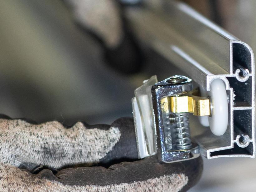
Bottom track uses rollers with springs. Springs push rollers upwards
