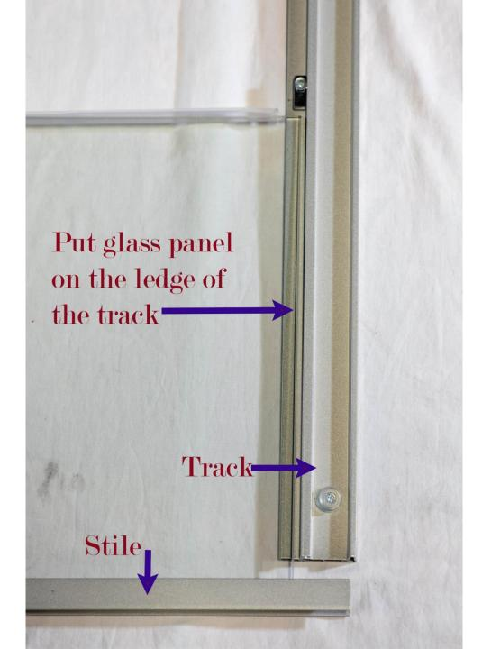
Put screw through pre-drilled hole on stile and go into screw hole in track
