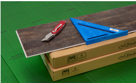
Cutting boards using Score and Snap technique
