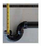
6. Slide the Drop-In Drain on the ABS or PVC 1 ½" pipe making sure it sits flat on the floor
