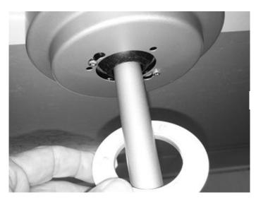
Photo 7: Key holes on the bottom of the hanger cover.
