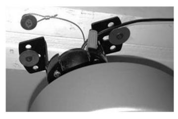
Photo 5: Safety cable attached near hanger
