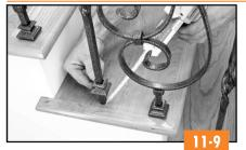
Finish the installation by using epoxy to fill any void around the base of the baluster and to secure the base collar.
