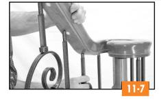
Working one baluster at a time, place the rail system on top of the balusters and install the rail permanently to the newels. Each baluster should then be rotated one turn to assure even coverage of the epoxy.
