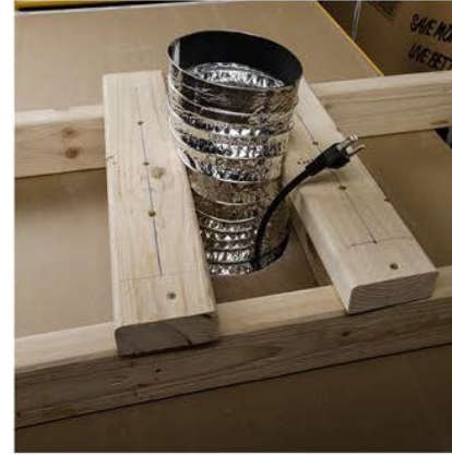
19. Secure the duct to the damper/air flapper with HVAC foil tape (as pictured) or duct tape.
