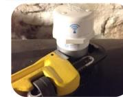
Use the pipe wrench on the metal body of the device to tighten. Do not use the pipe wrench on the cap.
