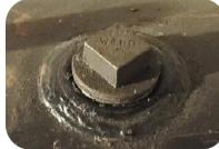
Locate one of the unused openings on the top of the tank. Use the pipe wrench to remove the plug. For dual tank setups with one fill pipe, install the gauge in the vented tank. Apply thread sealant (pipe dope) to the bottom threads, and thread gauge in by hand.
