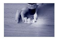
Pre-drill a hole in the floor with the correct drill bit. See above instructions.
