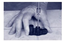
Once you find the joists, focus on the spot on the joist where the movement and squeaks are coming from. Then drive the screw through the shorter opening in the fixture.
