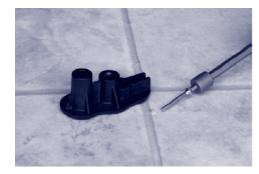
The screw is now set <sup>1</sup>/<sub>5</sub> of an inch below the floor. Take a hammer and tap the small bump that is left to smooth out the hole and force the hole to fill over.
