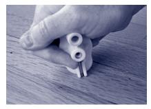
Rock the fixture back and forth until the head of the screw snaps at the score.
