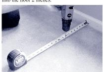
**Step 4.** Shift the drill into reverse. If the screw doesn't back out, the threads of the screw aren't in the joist. Lift the drill while you slowly reverse the drill, this will back the screw out. Move over an inch, moving away from the wall or the vent if you are using that, and drive it down again.
