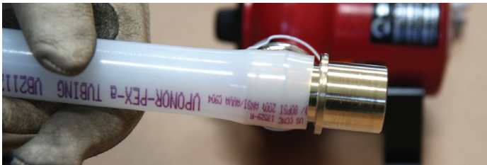
Figure 21: Heat Connection
