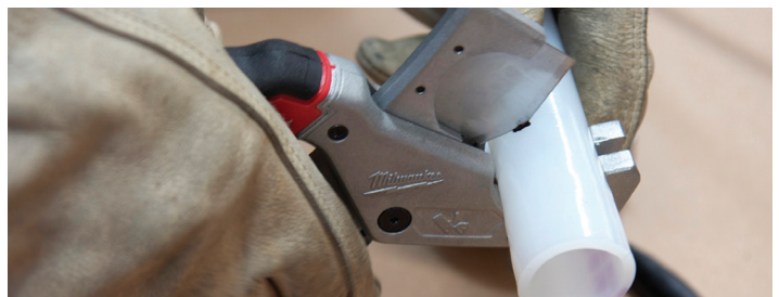
Figure 25: Cut Pipe at Marking
