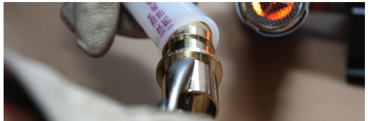
Figure 22: Work Piping Back and Forth
