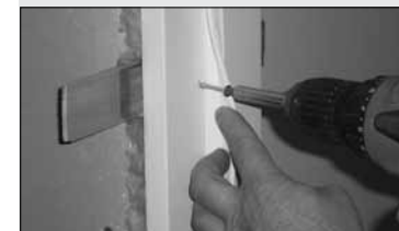
Figure 11: Screws are installed through the jamb, shims and into the 2x wood studs or bucking.
