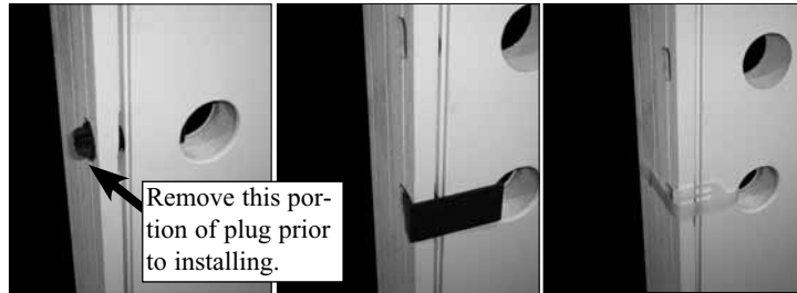
Figure 5: Some door units may be supplied with a "clip" or "plug" holding the panel aligned and closed during the initial installation steps. Do not remove at this time. Some door units may be supplied with a double headed nail or screw holding panel closed - this needs to be removed at this time.
