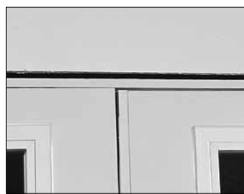
Figure 18: The gap between the door slabs and the head is not evenly aligned.
