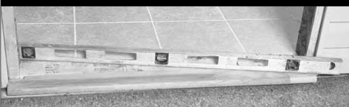
Figure 1: A clean, level, solid sub-floor area is essential for successful installation.
