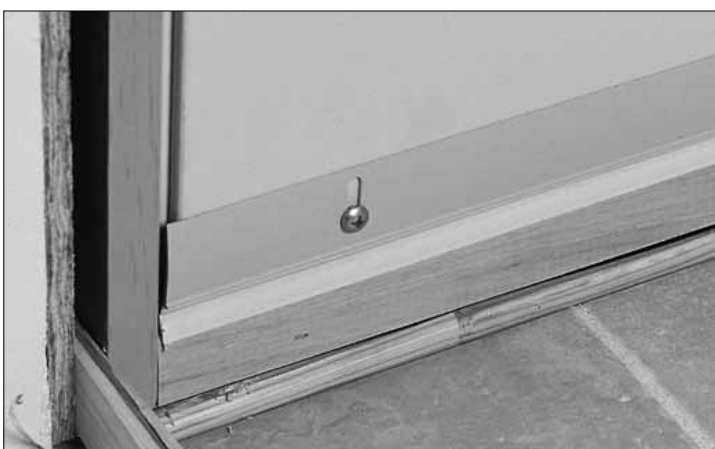
Figure 34: U-channel sweeps are adjusted to form a tight seal with the sill.
