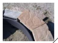
**Step 5**: Install the caps (12 units). Place the first top cap directly over one of the blocks in the second course allowing the cap to overhang the front of the block by about 1.5". Continue around the circle making slight adjustments as needed so that the edges of the caps fit tightly in the circle. Once the caps are in place remove them one by one and glue as above. Install clean porous rock or gravel between the steel ring and the blocks.
