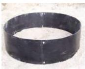
**Step 4**: Assemble the steel ring. Place the ring on the ground and using the bolts provided, bolt the two sides of the ring together. Install approximately 2" of clean porous rock or gravel inside the fire pit. Set the ring in the center of the blocks. Once the ring and blocks are all in place remove one block at a time from the top course and glue to the two blocks below using a quarter sized dab of concrete adhesive.
