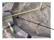
**Step 1**: Level the pad. Level a 70" circular area of gravel or rock on compacted soil with the top of the pad being 1" below grade.
