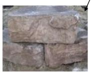
**Step 3**: Install second row of blocks (12 units). Place the first block on top of the bottom block staggering the intersection of two blocks on the row below. Continue around the circle making slight adjustments as needed so that the edge of the blocks fit tightly in the circle.
