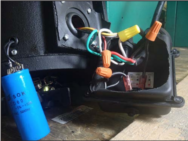
Figure 60. Main motor and capacitor (110V).
