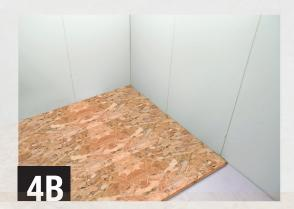
Install one of the recommended underlayment substrates below directly on top of DRICORE Insul-Armor.
