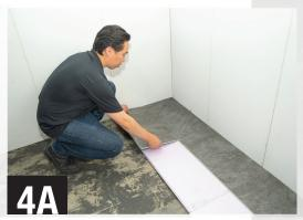
Once the first row of DRICORE Insul-Armor is installed, we recommend laying your choice of hard surface floors immediately on the newly installed row of Insul-Armor (reference Installation Hint #1 for details). We will address carpet installations in the carpet section.
