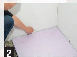
Start with a full panel with the grooved edges against the finished walls. Leave a 1/4" of space (for expansion) on rooms less than 20' long, and 1/2" for rooms longer than 20'.
