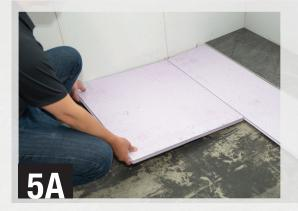
Work your way across the room installing one row at a time of the DRICORE Insul-Armor panels, then the finished floor treatment, until the room is complete. Remember to stagger the joints of the DRICORE Insul-Armor panels sufficiently row to row. Also, always follow the installation instructions of the finished floor as recommended by the manufacturer. Pay attention to acclimation requirements, and spacing at the room perimeter for expansion.
