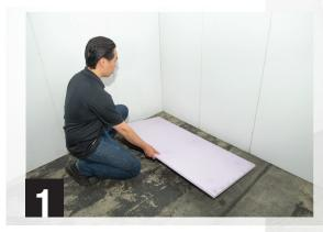
While you can lay the DRICORE Insul-Armor panels in either direction, it is generally laid with the 4' length running the longest dimension of the room.
