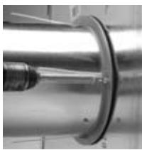
**Attach flex duct with zip tie or metal duct pipe with sheet metal screws.**
