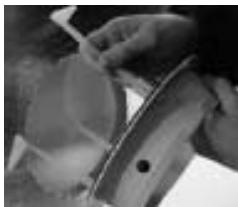
**Remove Gasket “Cover” from back of Take Off. Insert Zips with the “hook” faced away from the center and entering the zip clip holder from the back toward the front**
