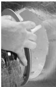
**If using the damper version make sure the damper handle or screw driver slot is on the right side of the take off and the damper, when open lies horizontally**
