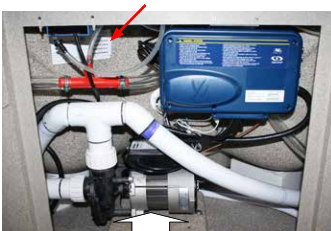
110 Volt Equipment Compartment
