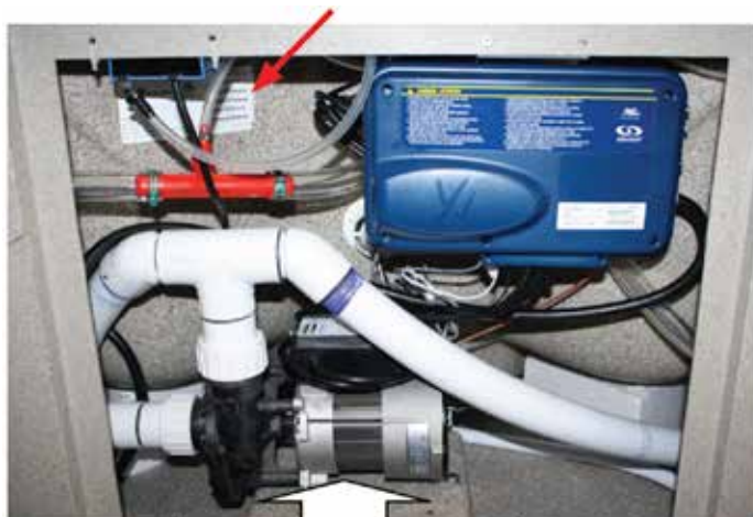
110 volts Bloc technique
