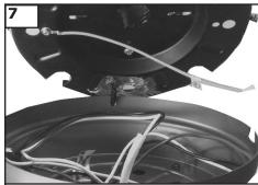
Carefully lift the fan motor assembly and engage the slot in the motor housing with the hook on the mounting plate so that the motor is securely suspended.
