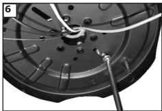
Securely attached the mounting plate to the outlet box using two screws supplied by the outlet box. Use metal outlet box suitable for fan support (must support 35 lbs).
