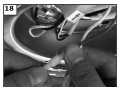
Connect white wire from fan to white wire from light fixture. Then plug blue wire from fan to black wire from light fixture.
