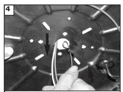
Thread safety cable through center hole of the mounting plate. Thread your house wires through center hole also. These will be needed for wiring of the fan.
