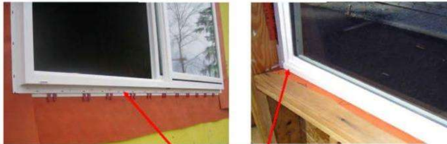
Sloped Sill Pan™ Installation Detail
