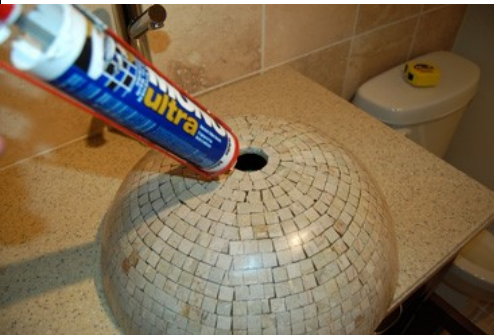
Above: Process for "Above Counter Mounting"
