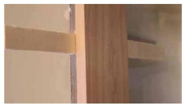
If installing a flush mount in-swing door, check both sides of your rough opening and start with the side that is the most level. Using the supplied screws, secure door jamb to opening. Use shims if necessary to keep the jamb level and plumb.
