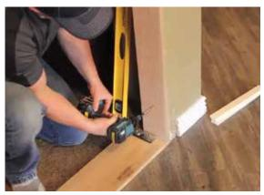
If you are installing a flush mount out-swing door, the non-hinge side of the jamb will be visible when the door is in the opened position. As such it is preferable to attach the jamb directly to the rough opening on that side. You will need to check to be sure that it is very level and if it is not it will be necessary to use shims.
