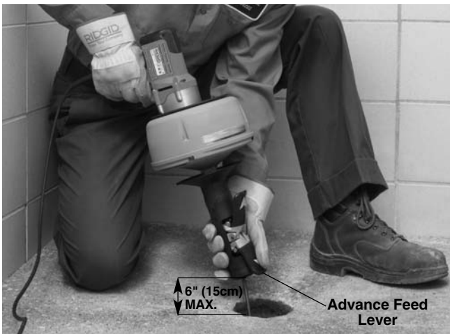
Figure 10 – Feeding Cable With AUTOFEED
