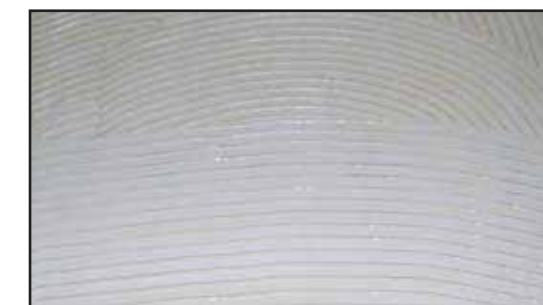
Example of properly troweled adhesive application
