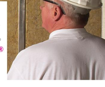
Thermafiber® Fire & Sound Guard® Plus is a hybrid light-density mineral wool batt that is designed to use in both interior and exterior wall cavities. This product combines the attributes of Thermafiber® UltraBatt™ and Thermafiber® Fire & Sound Guard® into one product, saving time for the installer.
