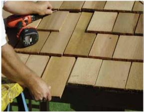
**46.** Roof **Filler Shingles** are included to cover roof seams. Starting at the bottom, slide the first Long Shingle in until flush with other bottom shingles.
