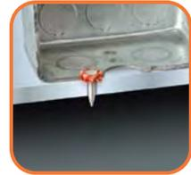
Choose a pin that is long enough to penetrate at least 1" into concrete and at least 3/16" **through** steel.
