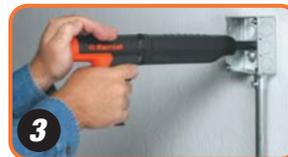
3 Press the tool firmly against the item you want to fasten, compressing the barrel. Pull the trigger to fire the tool.
