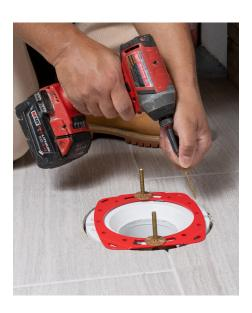
Do not wipe excess silicone off until the repair ring has been secured to the subfloor.
