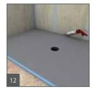
Set up a continuous 1/2" (12.7 mm) bead of wedi Joint Sealant along the pans channel on the outer perimeter and only in areas where you can immediately install a wedi Building Panel into the fresh sealant.
