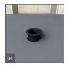
Drop the drain body firmly into the sealant.
