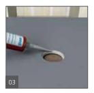
Set up a continuous 1/4" (6.4 mm) bead of wedi sealant along the top side of the wedi Fundos' valve groove profile. Optionally you can apply the bead on the underside of the main drain body's flange. This will help keeping sealant off the threads of the main drain body when it is inserted.
