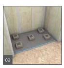
Press the Fundo firmly into the thinset bed, ensuring that the installation is level and void free. Apply some weight equally and leave on surface and drain area to allow the thinset to initially cure without being disturbed (e.g. thinset bags).
