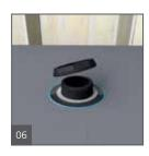
Tighten the gaskets firmly to the bases' steel ring using the locking nut. Make sure the drain body is still safely received in the valve-bead of sealant. Smooth out excess sealant over the drain body's flange surface.
