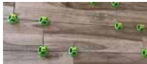
Large format Tile floor Install
