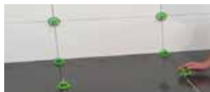
Floor & Wall Tile Install
