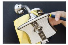
With the cloth fully covering the connection, use pliers to further tighten. Be careful not to mar the surface of the shower head with the pliers.
