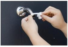
Apply the included Teflon tape by wrapping it around the shower arm threads a few times.
