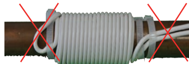
Example of wrong wrapping
