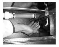
Position the hose clamp into position then connect the tube to the PVC pipe coming out from the bottom of the mirrored glass panel.
