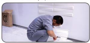
5) Using the knife to cut panels easily when meet corner or circuit of the wall.
