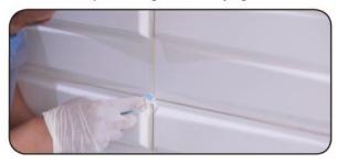
The water-based putty also can be used to repair the defect and holes of panels as well as the defect comes from installation.
