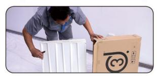
Open the box, put the panels on the floor for 24 hours to balance the moisture between the panel and the environment to prevent excessive expansion or contraction after installation.
