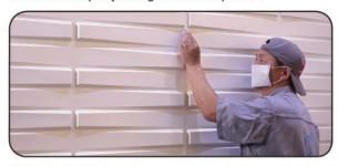
2) Normally it takes two hours to make the putty dry. Then using sandpaper (120-300MU) to polish the extra putty,and cleaning the seams with dry cloth to keep it smooth and flat. Fill it again with the putty when crack or with hole,and polish it again after drying.
