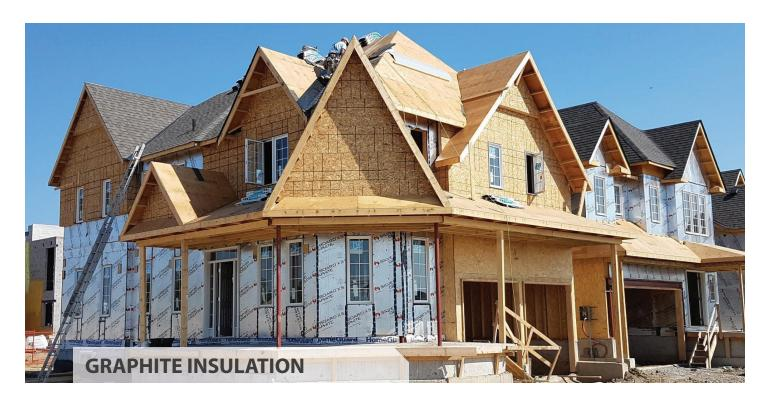
SilveRboard Graphite XS is a high performance, non-structural, rigid insulation board made from Expanded Polystyrene (EPS) with a layer of reflective metalized polypropylene film lamination on both sides.
