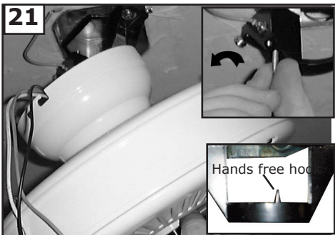
21 Remove the all thread studs from the lower part of the mounting bracket. Hang fan from mounting bracket by the hands free hook into a closed hole on the edge of the Canopy. Note: For Canadian mounting refer to Step #12.
