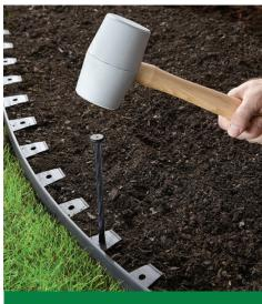
2 Use a rubber mallet to pound anchoring spikes through tabs to secure the edging. Pull the edging tight between spikes.
