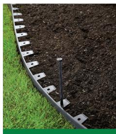
Clear the installation area of all grass, loose soil, mulch, and debris. Place edging on the cleared surface with anchoring tabs facing the planting bed.
