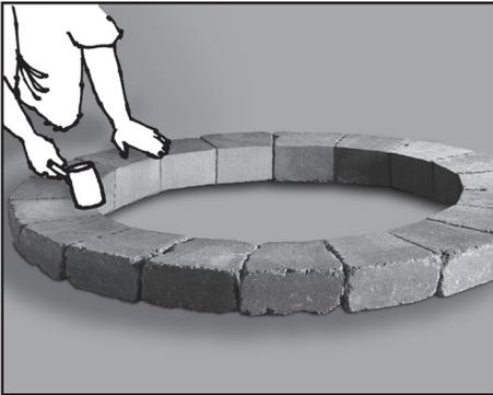
**4.** Place 19 wall block units on top of paver base. Lay them tightly together to form the circle. Level each stone front-to-back and side-to-side. Make sure each stone is even with the previously leveled block. Use a rubber mallet to level.
