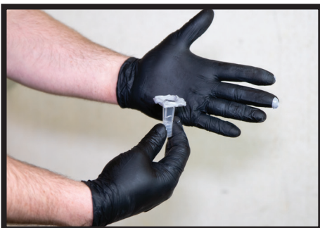
01: Roll the injection port in DRICORE™ PRO CONCRETE REPAIR CRACK PREP SURFACE PASTE
