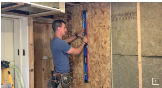
3. Determine if your installation will look best installed from the bottom up or the top down. Tip: thin cuts are usually best placed at the bottom.
