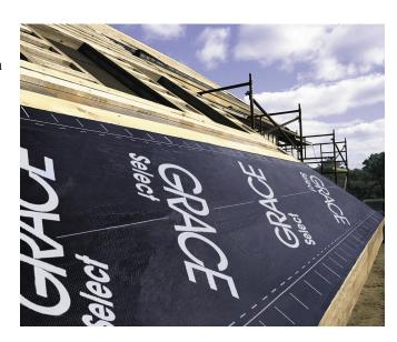
wind-driven rain from entering the structure. For wind-driven rain protection, full coverage with the membrane is recommended. Since Grace Select<sup>™</sup> membrane is a vapor barrier, the roof construction must allow for proper ventilation in full roof coverage applications.
