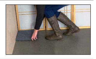
2. Keeping all additional tiles facing in the same direction, place tabs of new tiles over loops of already laid tiles and push down until they snap into place.
