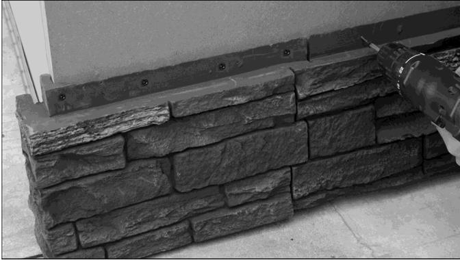
Slatestone panels have 8 unique panel configurations with a number, 1 through 8, molded into the back of the panel. Avoid racking the panels by placing like numbered panels next to or on top of each other.
