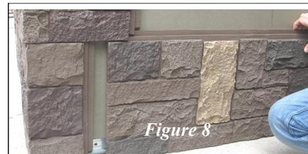
**Note:** There are 4 patterns of the Castle Rock Outside Corner. 2 Left patterns and 2 Right patterns. Check for the number on the inside of each corner. Corners are numbered 1 through 4. Alternate left and right corners with each course preventing pattern repetition.
