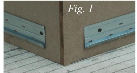
Optional: The panels can be face screwed at the bottom to eliminate the need for a starter strip. The screw heads will need to be caulked and painted for finished results. Paint Kit and caulk are sold separately.
