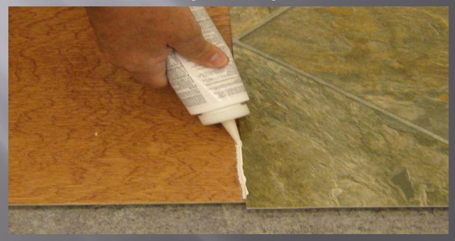
Apply S-761 Seam Adhesive continuously along the edge of the seam. **Do not** skip areas.
