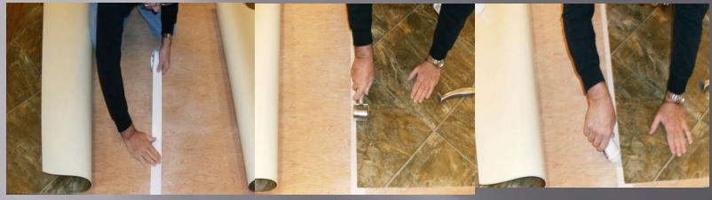
After seam is cut fold back and apply tape
