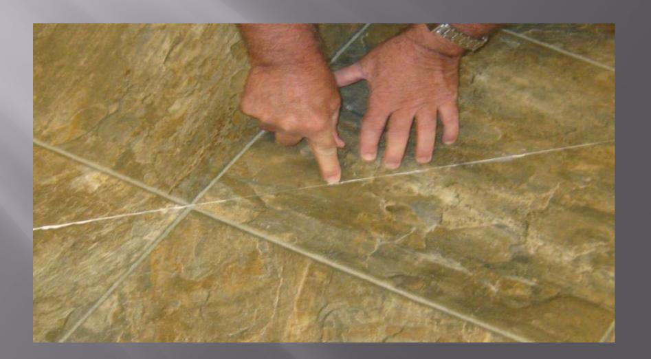
Excess S-761 seam adhesive will ooze to the surface of the seamed area.
