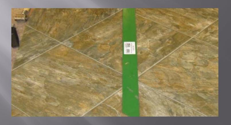
Hold the knife straight up and down double cutting through both pieces of material. If you are right handed the scrap piece you are cutting off should be to your right side.
