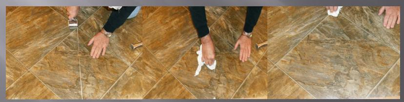
Lay in second piece and hand roll adhesive will ooze up between the pieces
