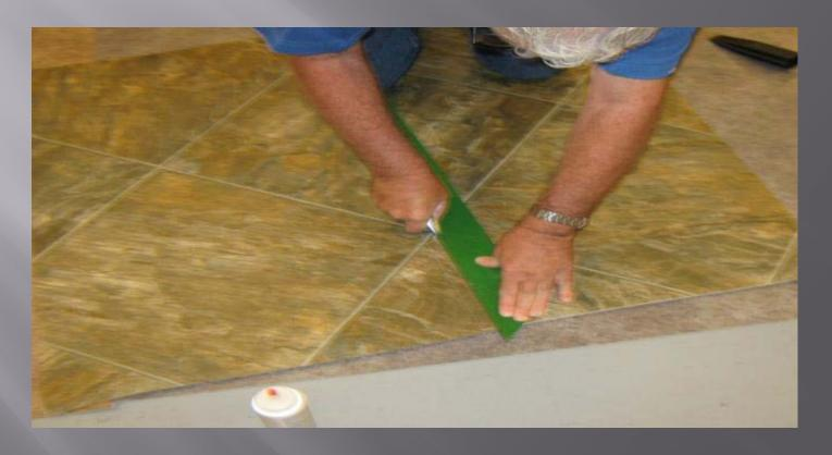
No matter which installation system you are doing seams are all cut the same, overlap and double cut
