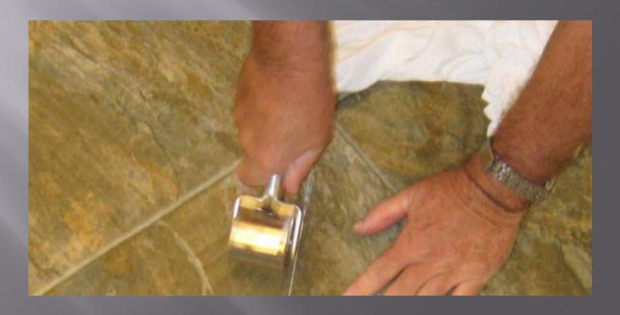
After completely rolling the seam, again clean the excess adhesive from this area with water and clean damp cloth. The new treatment is now completed. Roll the floor with 100 lb. roller when installed with adhesive(S-289, S-288 for the ToughGuard II Installation, Fiberglass Reinforced Sheet Flooring Installation or S-235 or S-254-for the Residential Feltbacked Installation) Do not roll material with 100lb roller when installed with the modified loose lay system.
