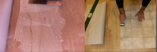
After cutting the seam fold back both pieces and apply adhesive using a regular notch trowel on porous and fine notch on non-porous substrates.
