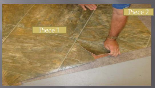
Place a 2"-3" wide piece of scrap under the area before the seam is cut. Place a straightedge in the area where you want to cut the seam.
