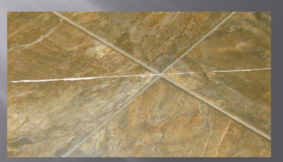
To clean the excess adhesive from the seamed area, use a clean cloth dampened with water.
