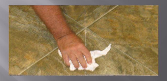
While rolling the seam, excess adhesive will ooze to the surface.
