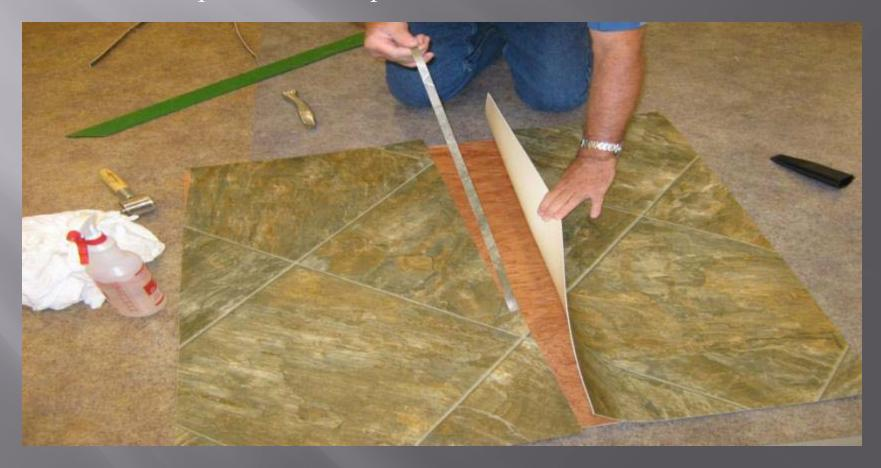
Fold back one piece from the S-289 adhesive and then apply a 1/8" bead S-761 Seam Adhesive on the edge of the other piece
