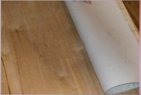
Apply adhesive either full spread or perimeter 12" band around the room. Do Not apply adhesive in the area of the seam Double cut seam dry.
