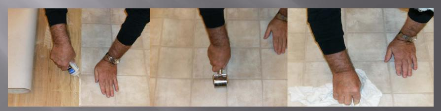
Apply a 1/8" bead of S-761 seam adhesive along the edge
