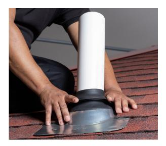
Press firmly to make sure the new rain collar sets on top of the existing rain collar to ensure silicone is completely compressed
