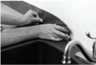
Place each section as if placing a puzzle piece
