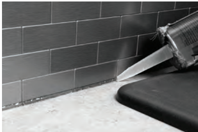
Caulking the countertop seam
