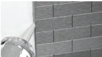
Finishing option 2: Caulking outside edges
