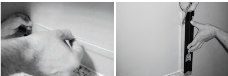
Mark horizontal and vertical reference points
