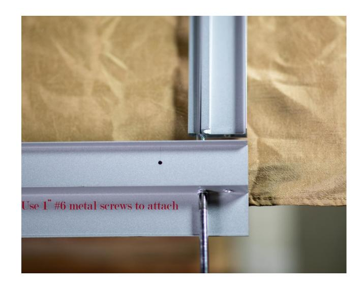
• Let screws go through pre-drilled holes on stile. The tips of the screws go into the screw holes in the track. Make a couple of turns to let screws stay in place.
