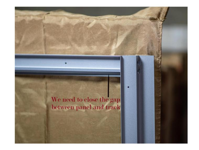
• We now ready to assemble the other track to the stile. However, we do notice a small gap between the glass panel and track. We need to close this gap. Use a rubber mallet to tap the end of stile while a person holding the other end of the panel.
