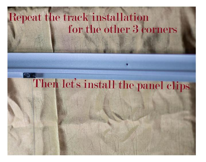
• Place panel clip onto the track ledge and in contact with glass panel as shown by this picture. Use 1/16" drill bit to drill a pilot hole on the first layer of the track. Do NOT drill both layers!!!
