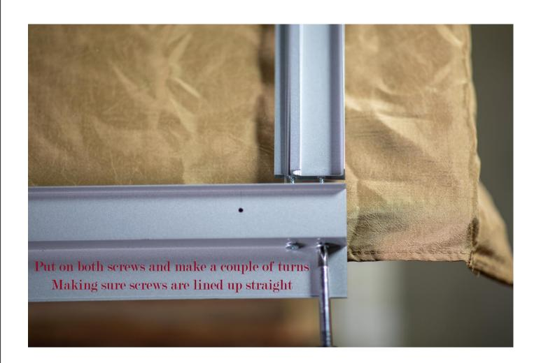
You can use hand or power driver to tighten the screws.
