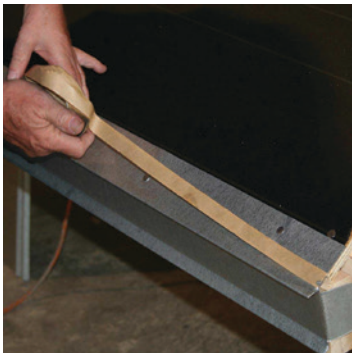
Gently unroll the butyl tape on the area to be sealed
