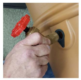
4. Square up the spigot or drain and carefully thread into the seal to avoid cross threading.
