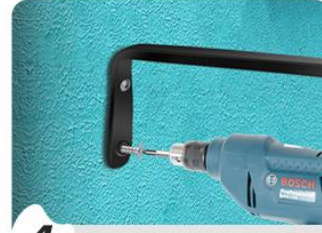
4 Install hooks with screws
