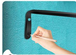
1 Mark the holes
