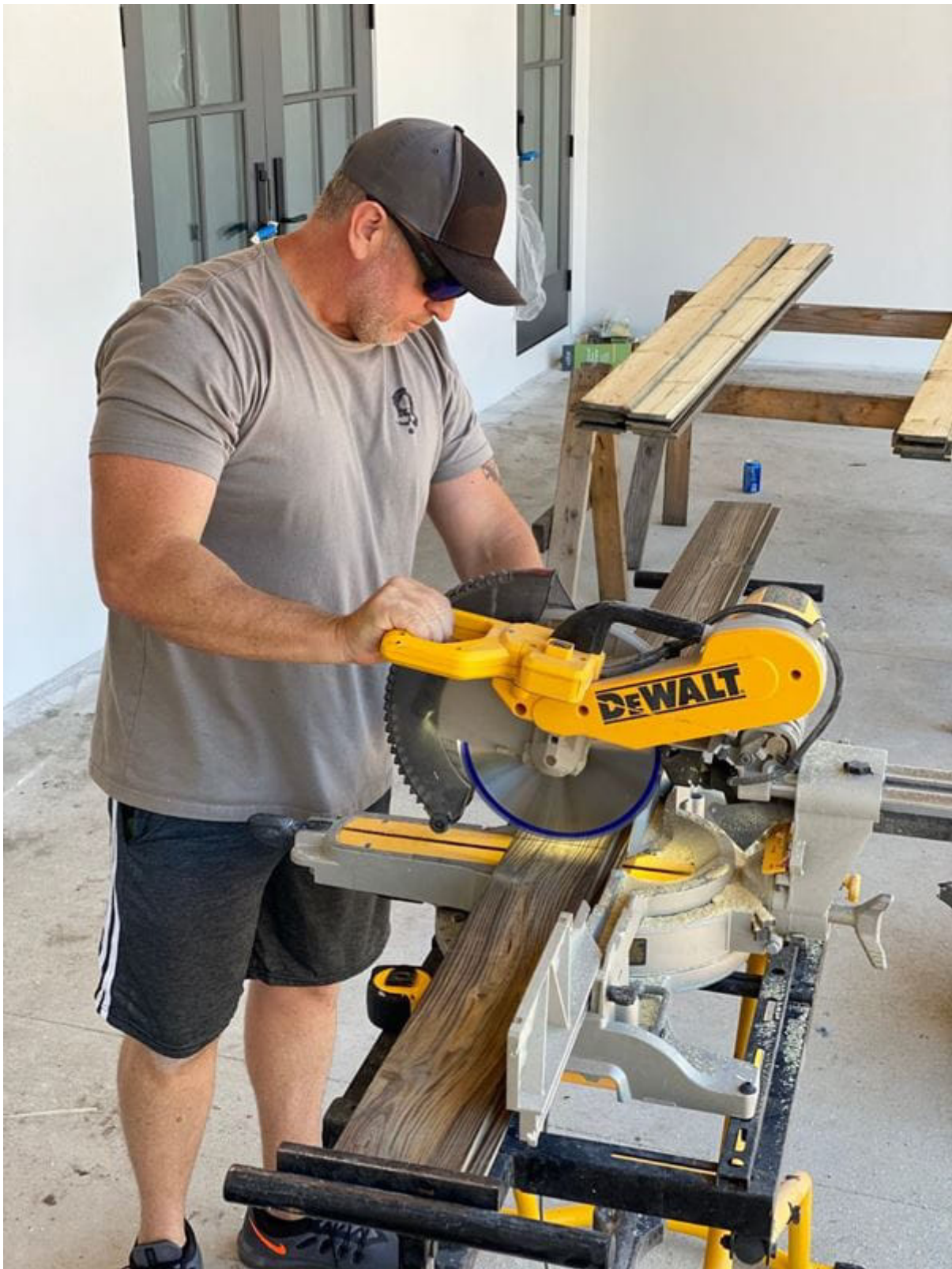
Jason using a chop saw to cut the shiplap.
