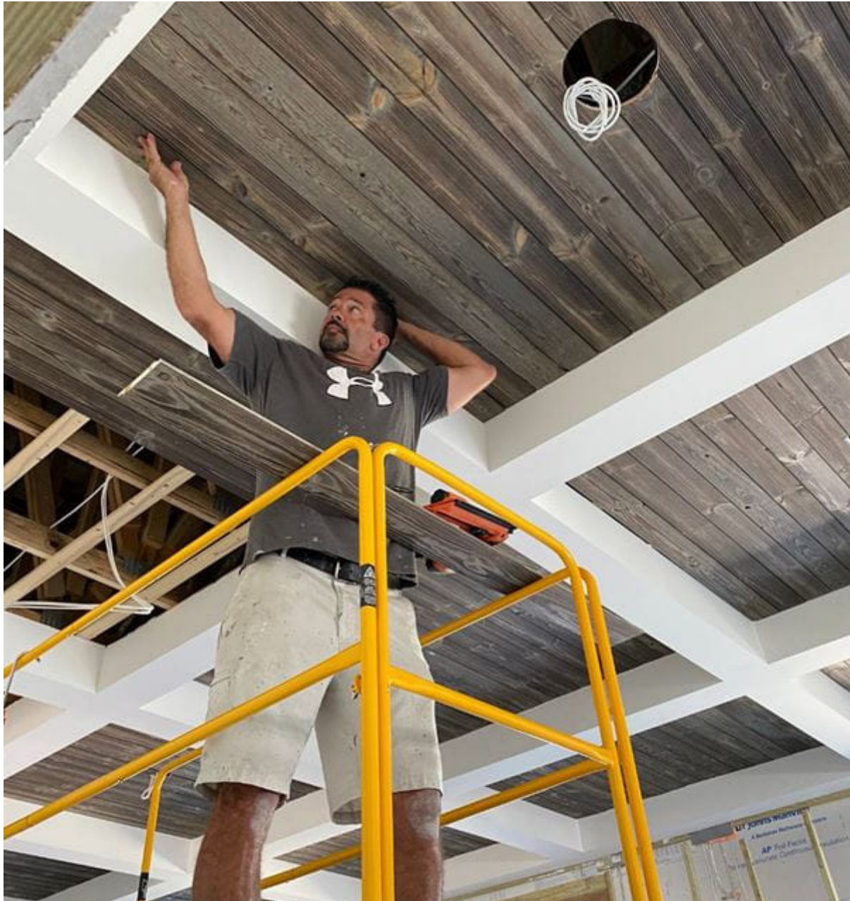
Doug installing the last rip board.
