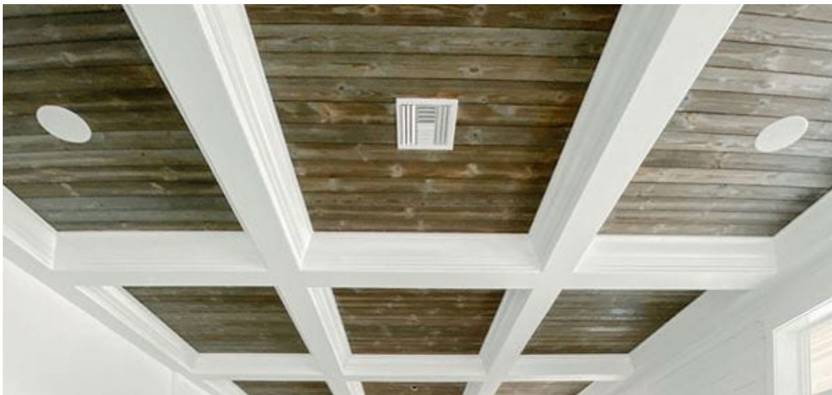
The ceiling took two days to complete.
