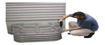
4. Mount clips to window well cover using bolts, and cap nuts provided. IMPORTANT! Put bolt through clip and cover. Secure using cap nut that has been provided (See diagram below).
