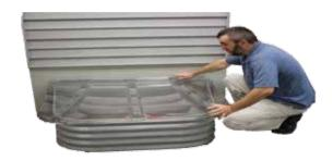
2. Mark position of holes for clips on center of well rim with a marker on the window well cover. Two(2) clips on each side and one (1) clip on the front of the well.
