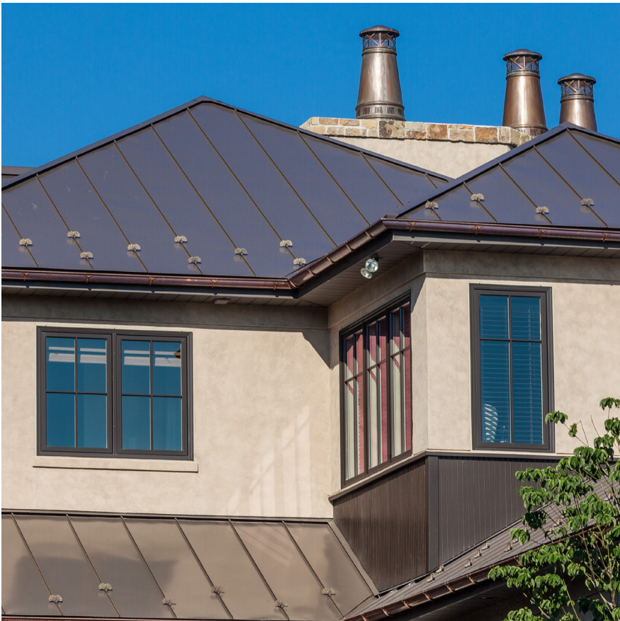
This home features a standing seam roof with Chimney Pot accents and a Snow Retention System.
