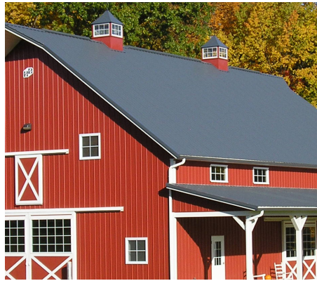
Grandrib 3 in Brick Red on the walls and Charcoal Gray on the roof create a classic American look on this barn.
