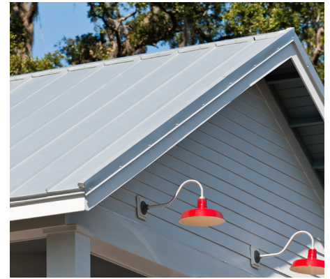
1 ½" SSR in Acrylic Coated Galvalume, selected for its reflective qualities, covers the roof of this home.
