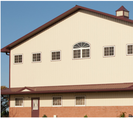
This building features Grandrib 3 Plus siding in Tan with a Grandrib 3 Plus Cocoa Brown roof.
