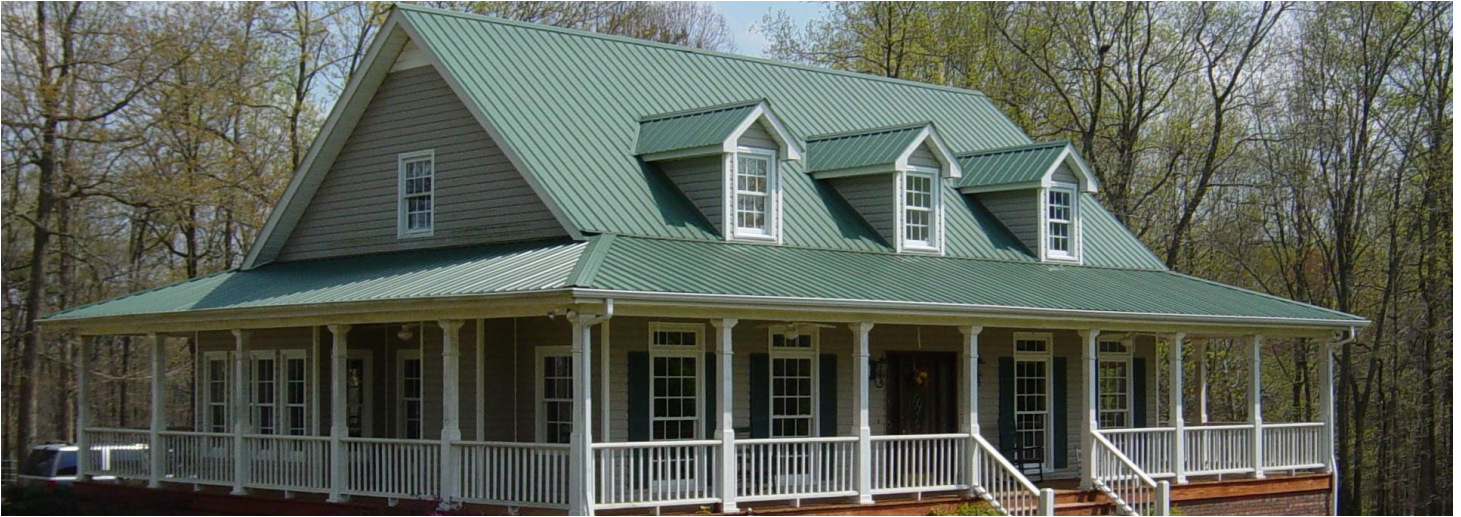
Grandrib 3 with Evergreen roof complete with gutter system.
