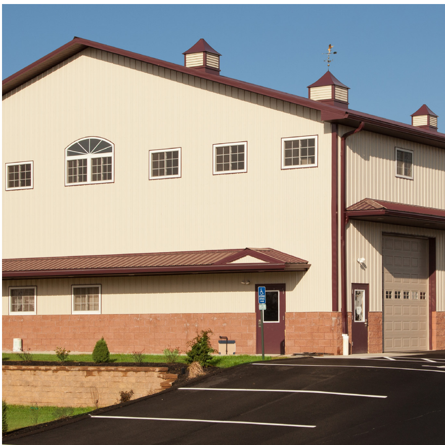
Project features Grandrib 3 Plus, aluminum soffit and cupolas.
